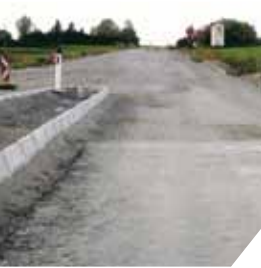
Reused for non-compacted load-bearing surfaces
